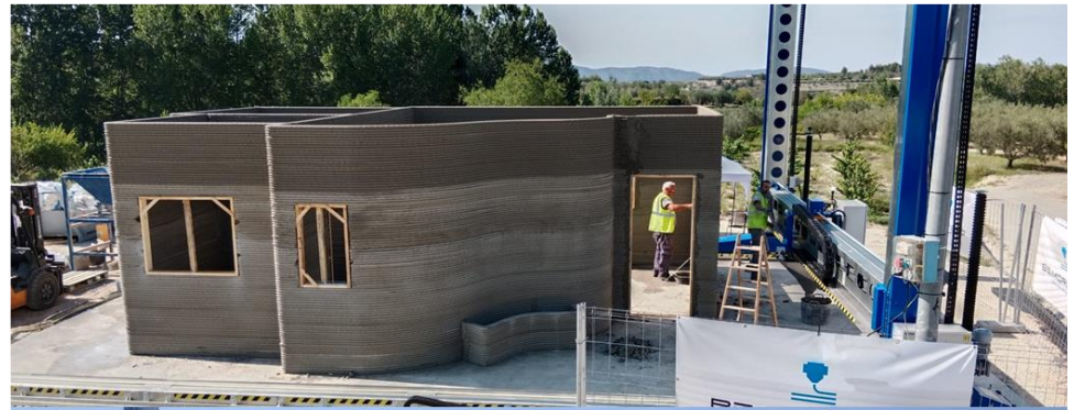
UBB-printer mounted in Valencia, Spain and 3d-printed house tested
