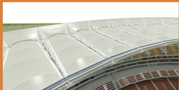
Figure F4 - Perth Stadium roof: An example of a modular structure with corrosion considerations
