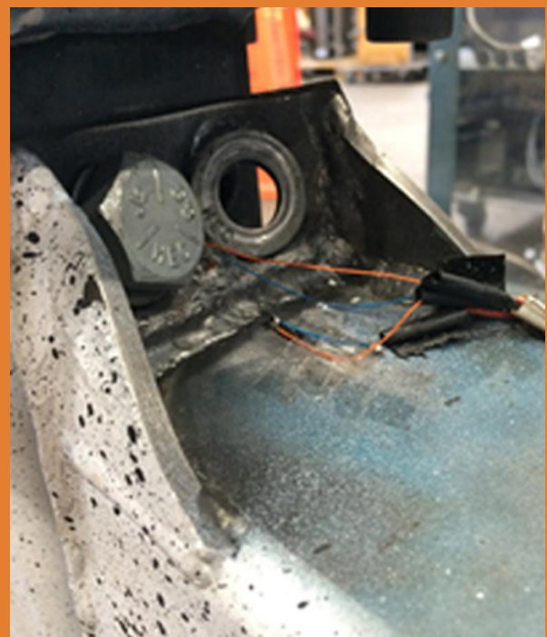
Figure A8 – Joint specimen with bolt fracture
