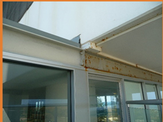
Figure F3 -Internal and external corrosion compared at Air on Broadbeach (Gold Coast, QLD). The protected façade has a markedly higher corrosive microclimate as rain does not clean off contaminants.
