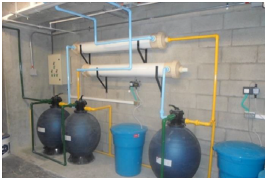
Figure 28: Grey water and rainwater treatment plants installed in the Biohotel
