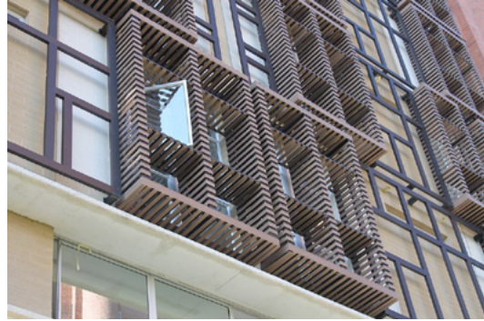
Figure 27: Building façade showing window elements designed for allowing natural light while avoiding sunshine income, thus providing energy efficiency and indoor comfort
