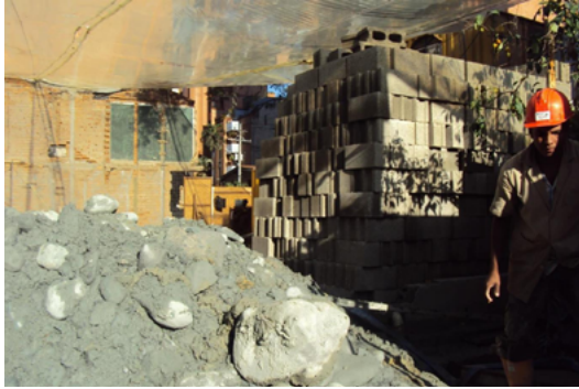
Figure 26: C&D waste from excavation and concrete blocks fabricated from it
