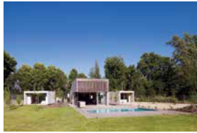
Finger Joint house Nogales, Chile
