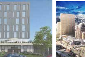
Origami Office Building Las Condes, Chile
