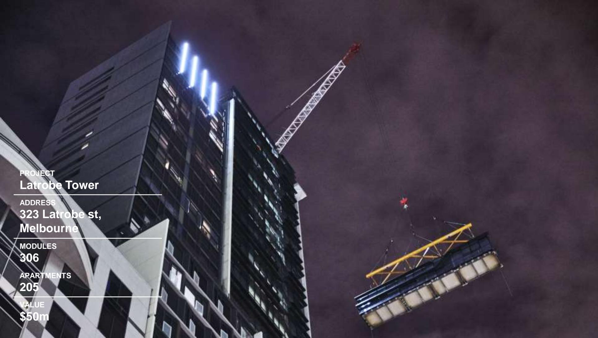
A low-angle, nighttime photograph of a tall, modern building under construction. The building's facade is dark with some windows illuminated. A large white crane is positioned on the roof, lifting a large, rectangular, blue and white prefabricated module. The sky is dark and cloudy. The overall scene is dramatic and industrial.
